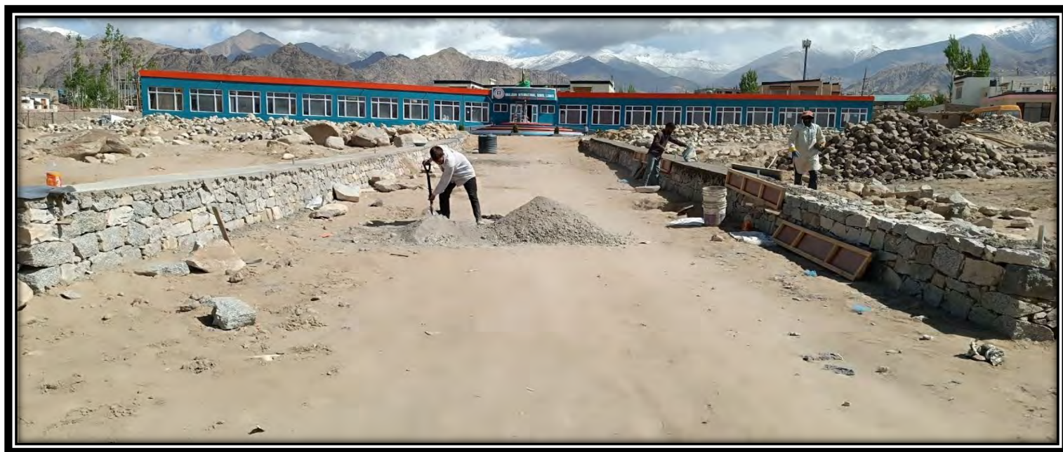
FIGURE 4: CEMENT COPING CONSTRUCTED ON BOTH SIDES OF THE ROAD'S SIDEWALLS TO ENHANCE STRUCTURAL STRENGTH.
