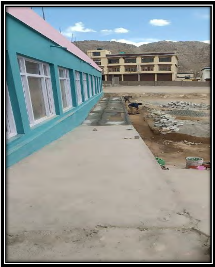
Fig. 5: Stone Pitching and Cement Concreting and curing of the Veranda
