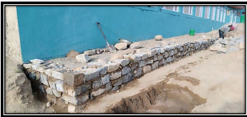
Fig. 4: Construction of Stone Retaining Wall for Veranda
