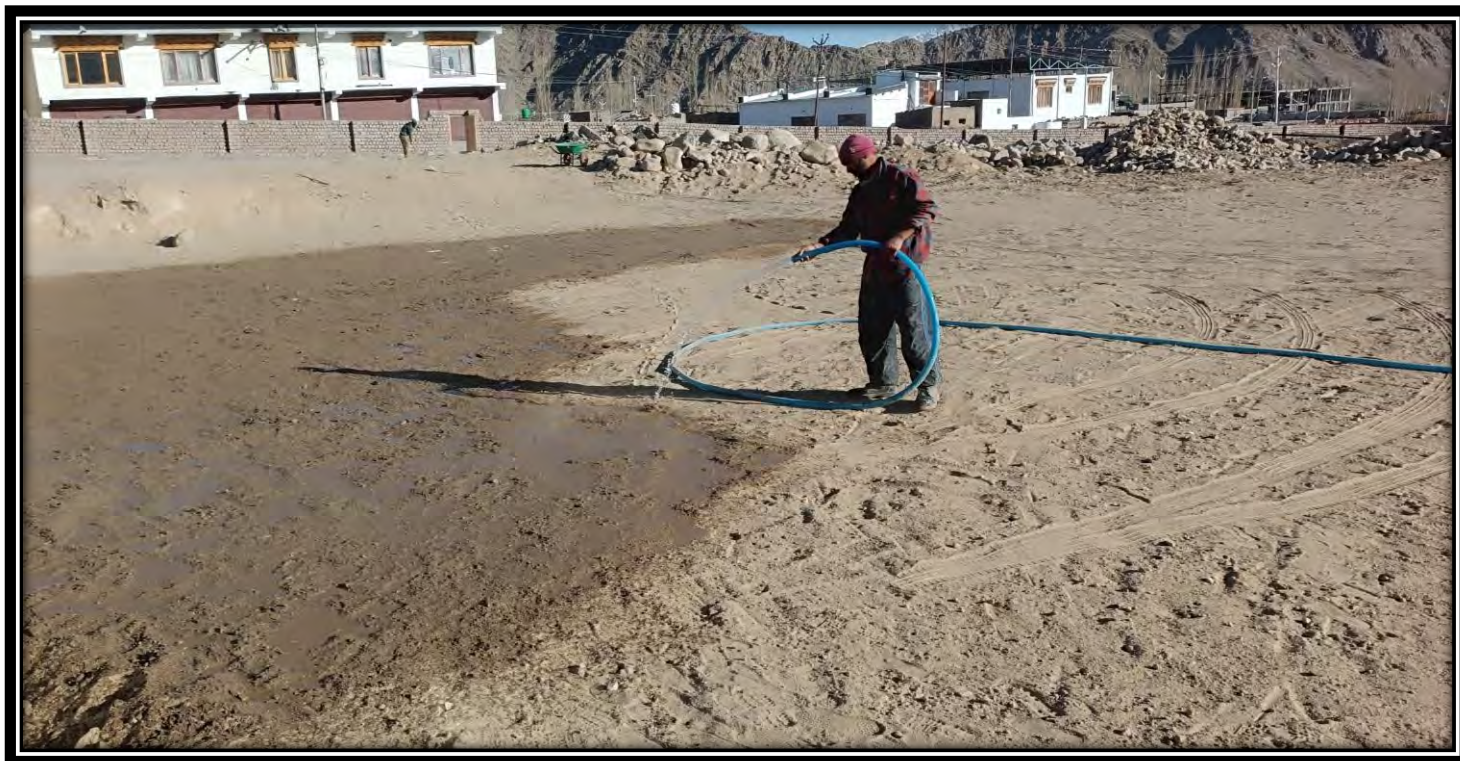
Fig-2: After levelling, a fine layer of soil was spread and moistened
