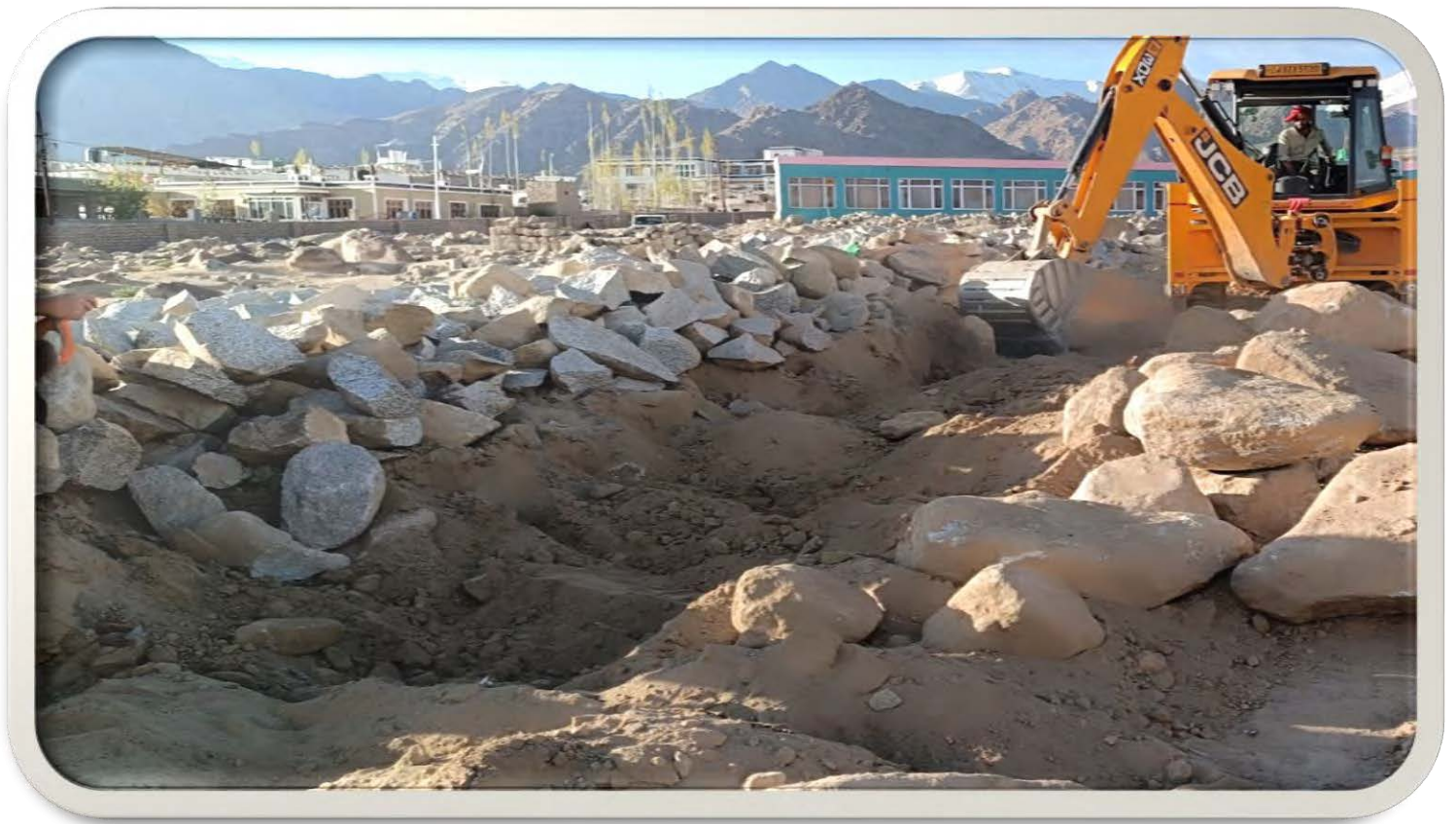
Figure 2: Boulders removed to prepare a leveled surface, followed by smoothing and grading..
