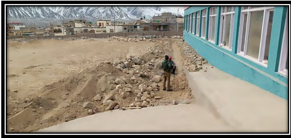
Fig. 2: Removal of Boulders and Stones for Veranda Construction
