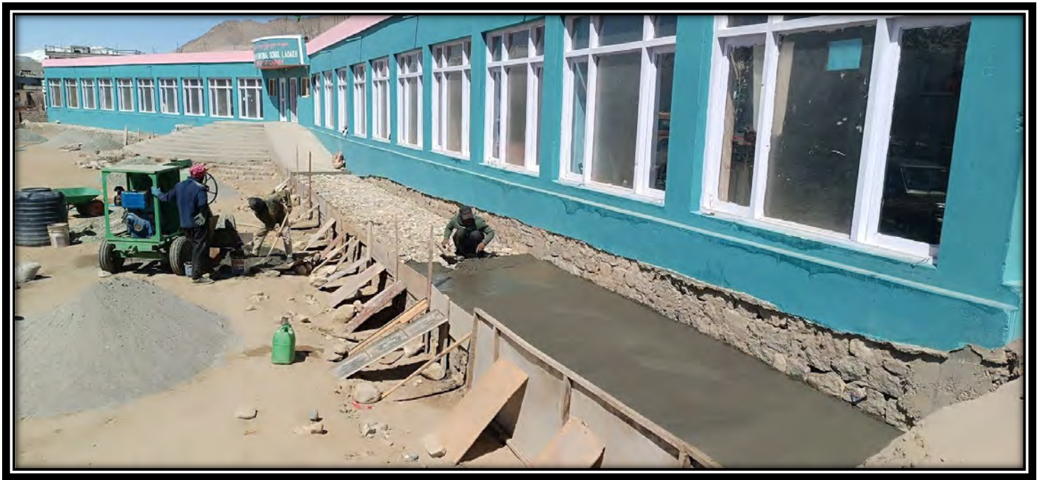
Fig. 5: Stone Pitching and Cement Concreting and curing of the Veranda
