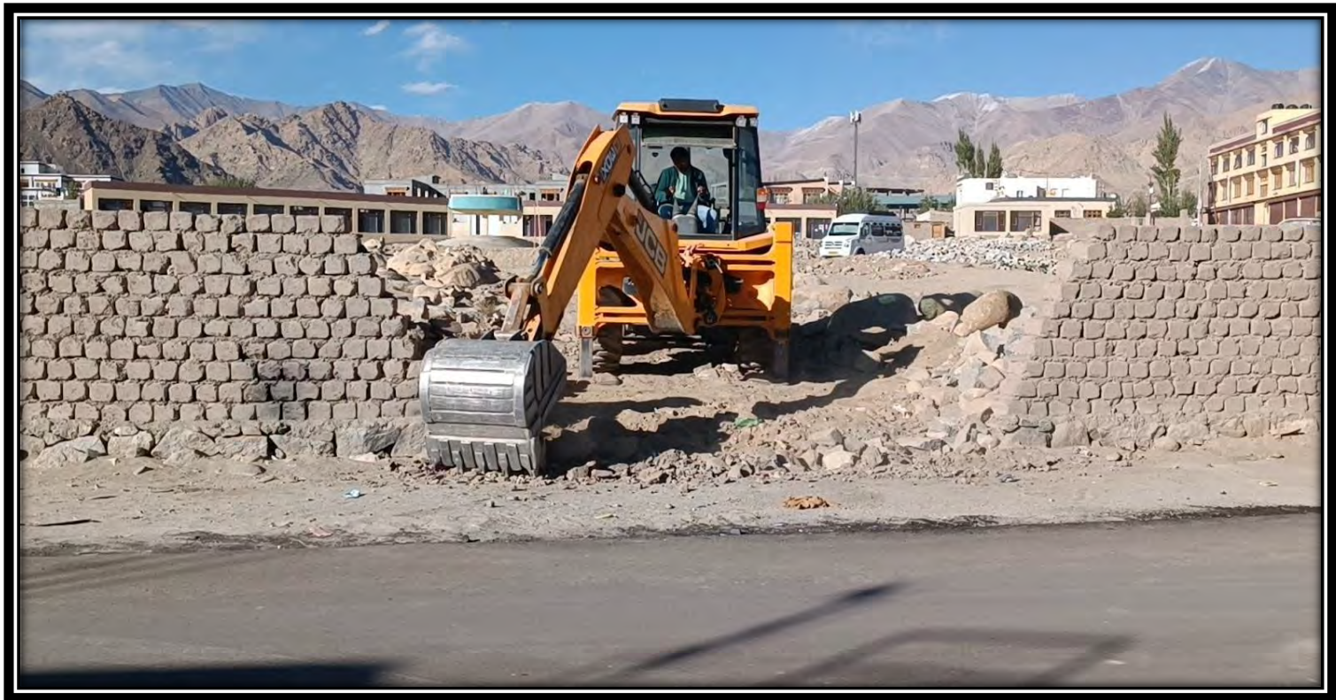
FIGURE 1-2: CONSTRUCTION OF THE ACCESS ROAD COMMENCING FROM THE MAIN ROAD, WITH ACTIVE INVOLVEMENT OF A JCB MACHINE AND LABORERS.
