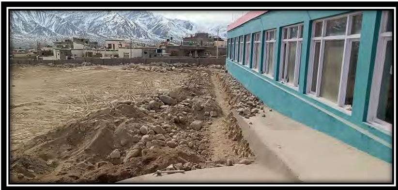
Fig. 1: Preparation of Foundation for the Veranda Construction
