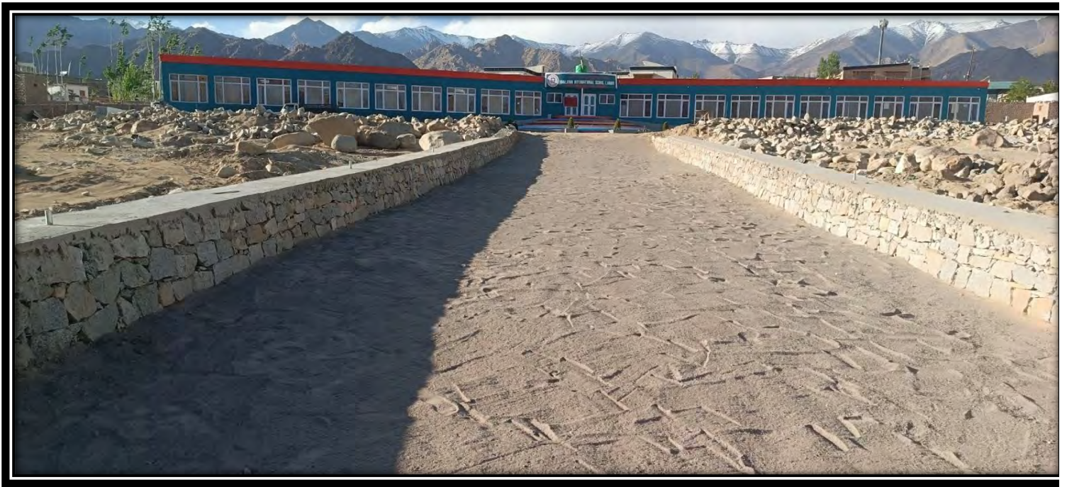
"Figure 4: Final layer of soil spread to ensure a smooth, compact, and stable road surface."
